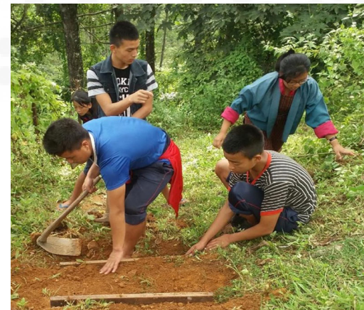
YCS students construct footpath to boys hostel.
